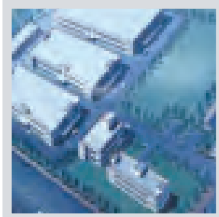
Wuxi Plant (China)
